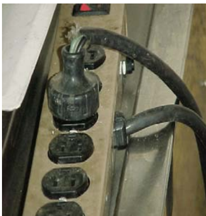
Fig. 3 Plug pulled from casing and insulation
